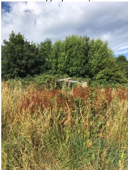
Abandoned plots with derelict structures
